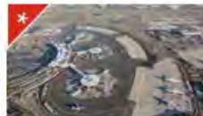
Newark Liberty International Airport Newark, NJ
